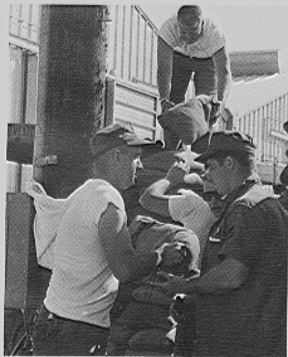
Building the walls
