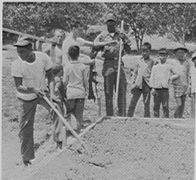
Cement is spread and smoothed
